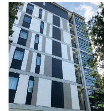
The opening of Haumarū Housing's new 41-unit development in Wilson Road, Glen Eden, is eagerly awaited by prospective tenants.
